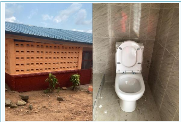
Figure 3: Before and after facility renovations
